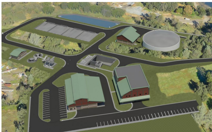
Rendering of PCWA's future Ophir Water Treatment Plant, a $227 million investment that will provide an initial 10 million gallons per day of treated water capacity and support long-term regional reliability.
